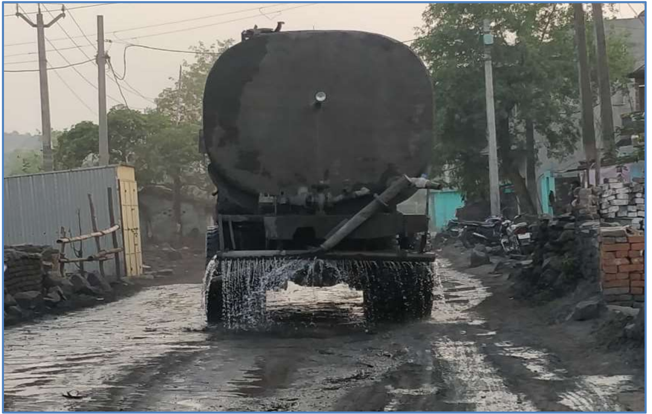
Picture 2 – Water Sprinkling on Transportation Road
