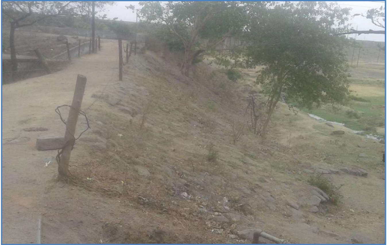
Picture 3 - Stone Pitching/embankment at Kari Jore
